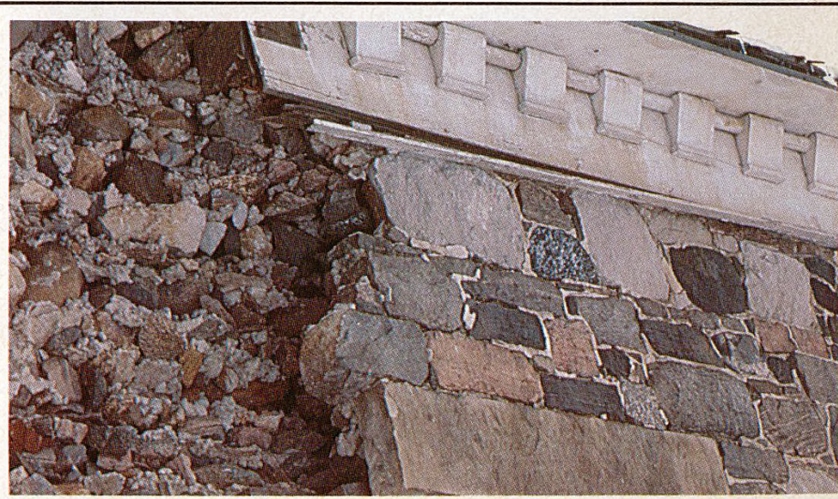
Exposed interior of a Stone Wall
