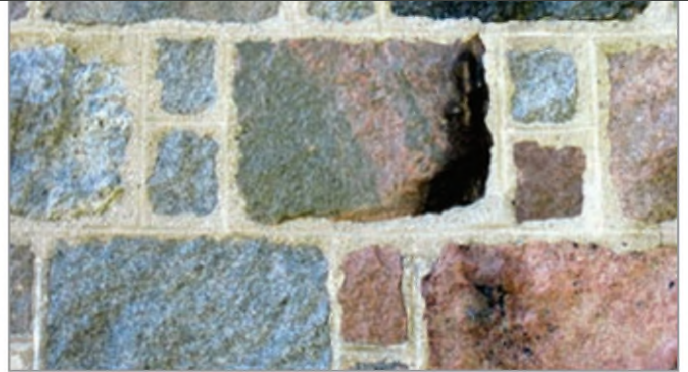
FIG. 17. CRELLIN'S ABERDEEN BOND STYLE MASONRY WITH 2 SNECKS, MCCOMB HOUSE, I 33 RD LINE, NO. 6603, NEAR HARRINGTON, OXFORD COUNTY. | KAREN E. ARMSTRONG.
